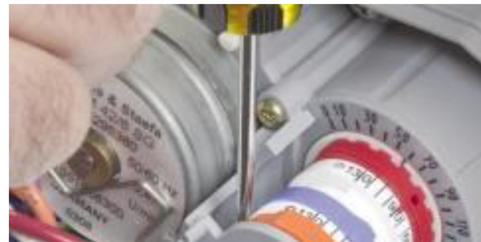
Transition Cam is set with Screwdriver
